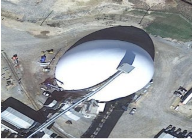
E-2 Plant Storage Dome
