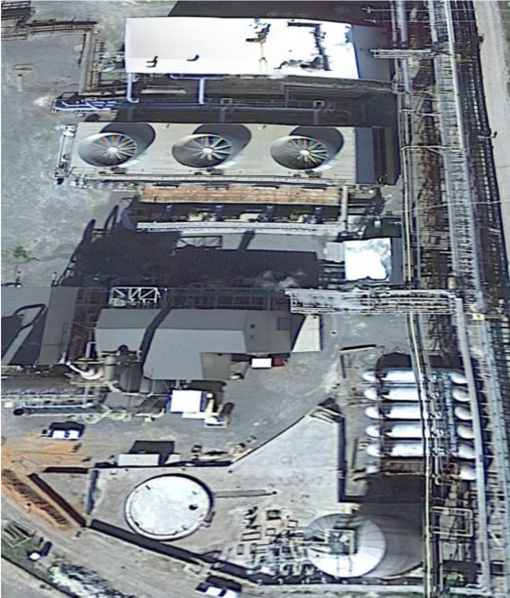
DMW #2 Nitric Acid Plant and Cooling Tower / New Boiler House
